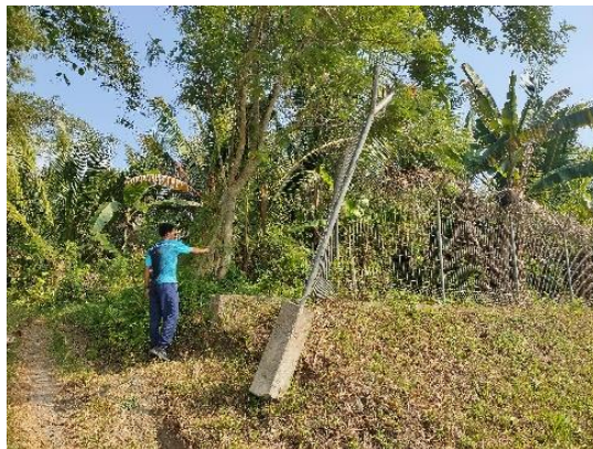
Gambar 3 Keadaan Parimeter Bandara Oesman Sadik
